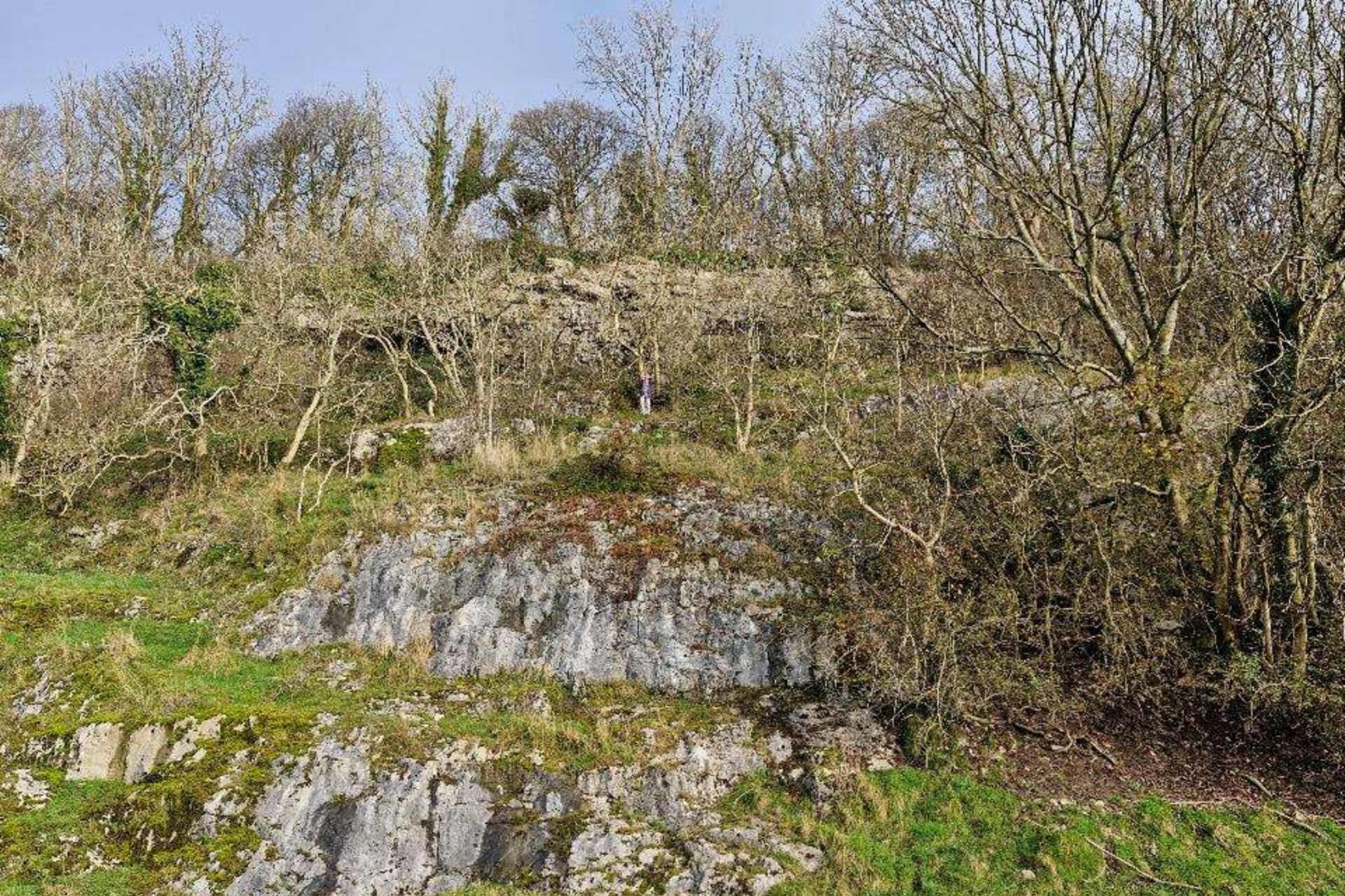
Archived LGS Head House Quarry, Cartmel. In a private garden, never visited since designated in 1993. Carolina is on the junction of Park Limestone below & Urswick Limestone above
